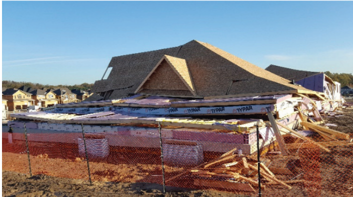
Figure 7: Wind damage to partially constructed homes in Waterloo (2017), Ontario. The image illustrates an intact roof resting on failed walls during construction.
